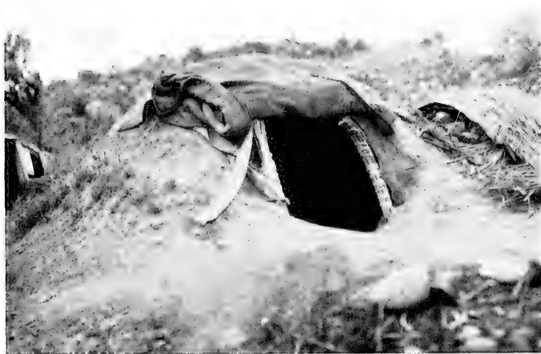
FIG. 191.—Shahaptian Indian sweat house built up of tulle reeds with matting of cat-tail rushes and covered over with earth. Still used by the Wanapum or Columbia River Indians. Located at the Lower Falls of the Yakima River, Benton County, Washington.
